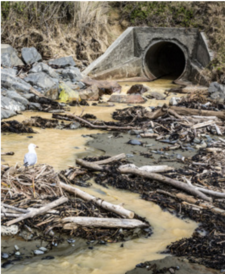
Stormwater outlet, Titahi Bay
